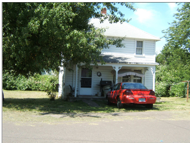
Northeast facade, looking southwest
