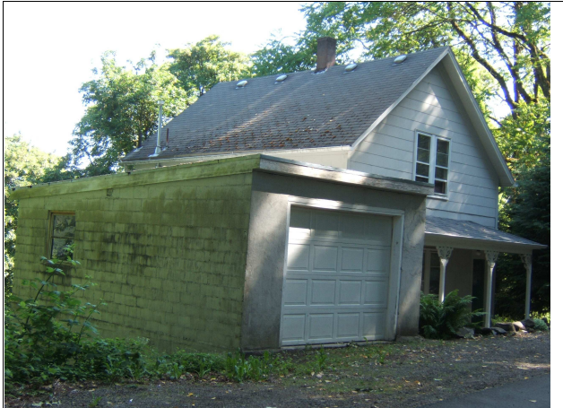
Southwest facade, looking northeast
