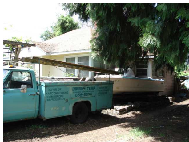
Southeast facade, looking northwest
