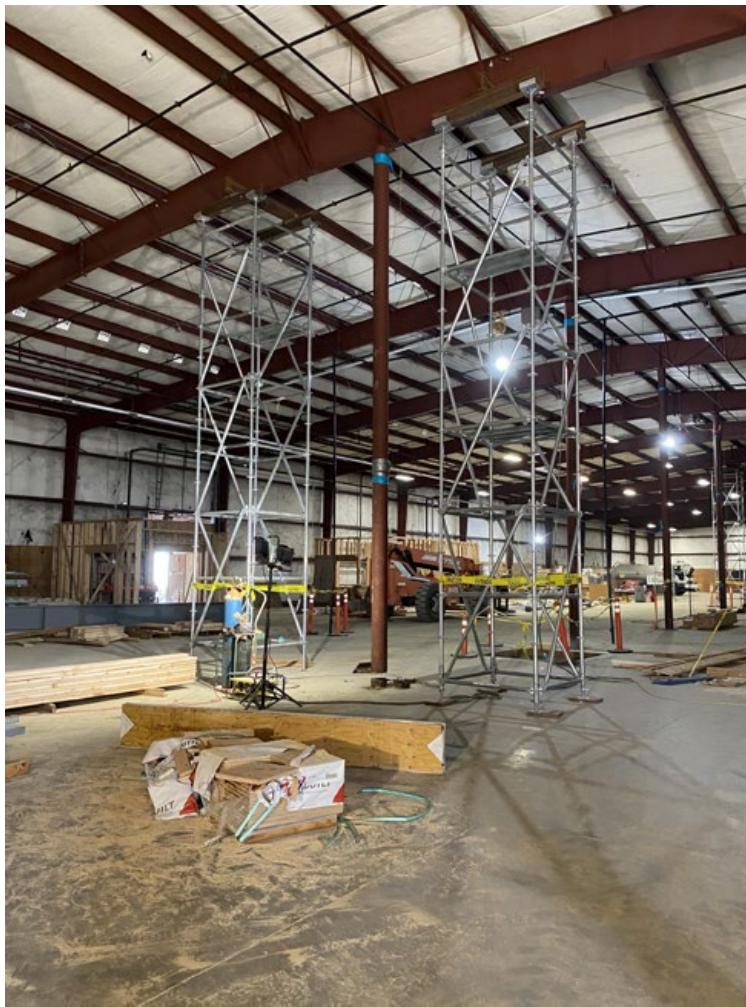
The structural upgrade of the existing building to a seismic level 4 presented challenges as well. The existing building consisted of tilt-up concrete construction, pre-engineered metal, wood framing, and light gauge steel framing from 6-7 additions or modifications over the life of the building—the result was a 75,000 sf puzzle. Scott Edwards Architecture performed comprehensive conditions assessments to understand all available upgrade options.
