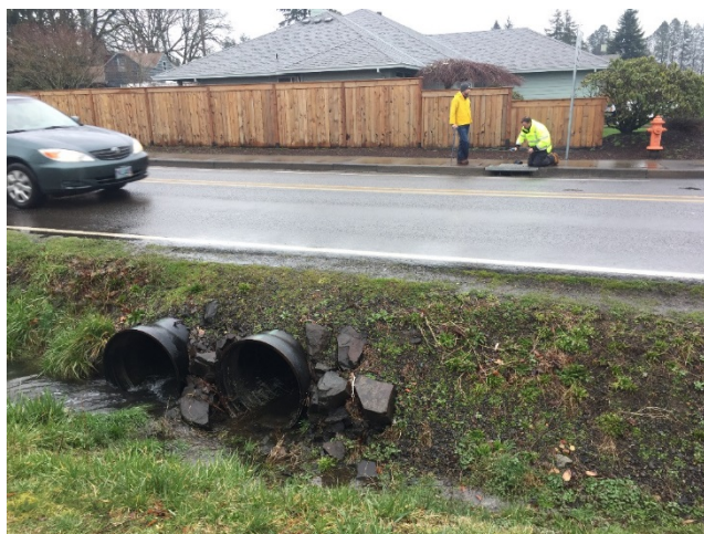
Figure 2: Inlet of culverts west of Leland Road
