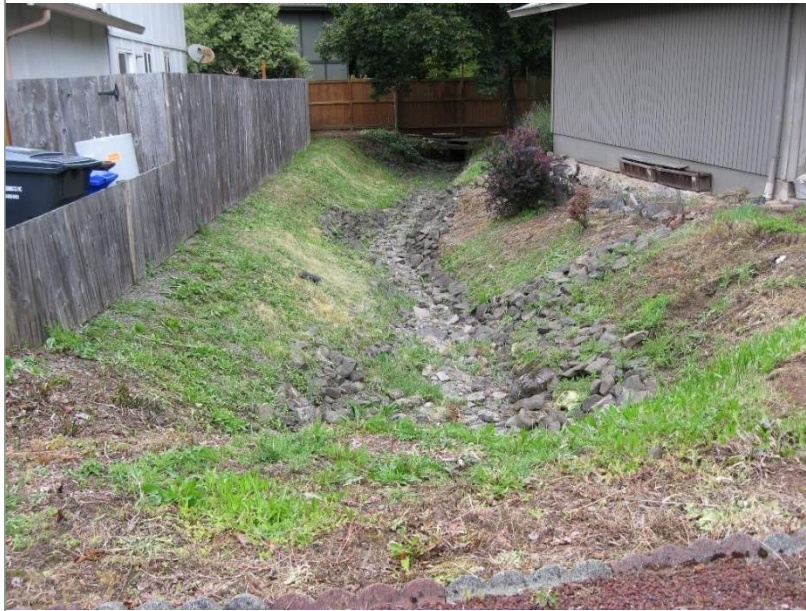
Site location: 205 Photo number: IMG_1574 Description: Open channel near 1013 Hazelwood Drive. Channel bed formed of large rocks. No incision/erosion.
