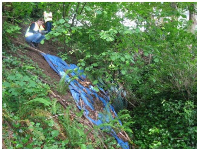
Image 2. Sloughing bank downstream of outfall location near Eluria Street
