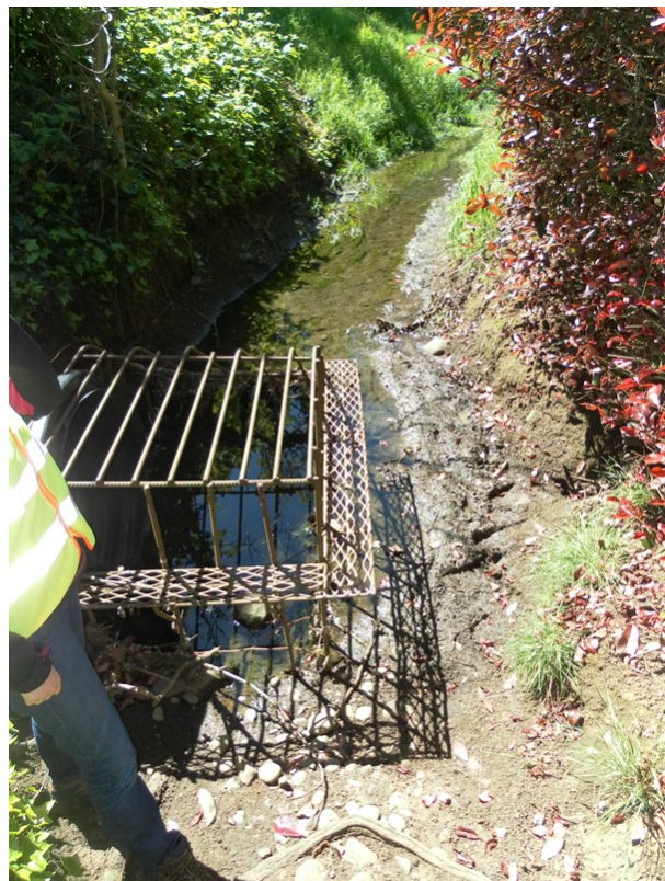
Inlet to culvert under Central Point Road on private property.
