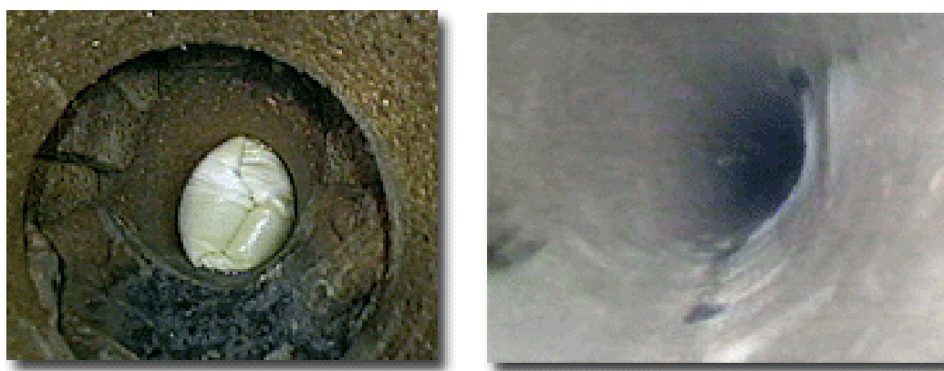
Figure G-6. Examples of cured-in-place point repair
