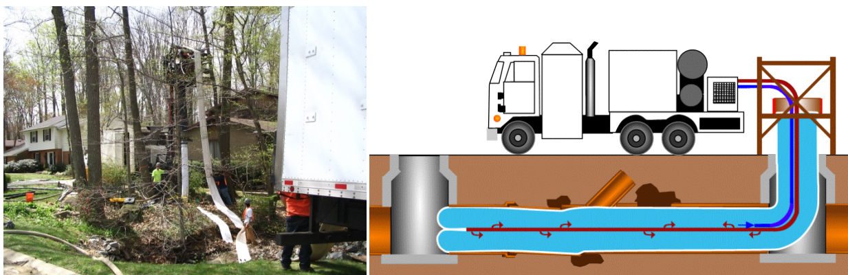
Figure G-1. Examples of CIPP installation
