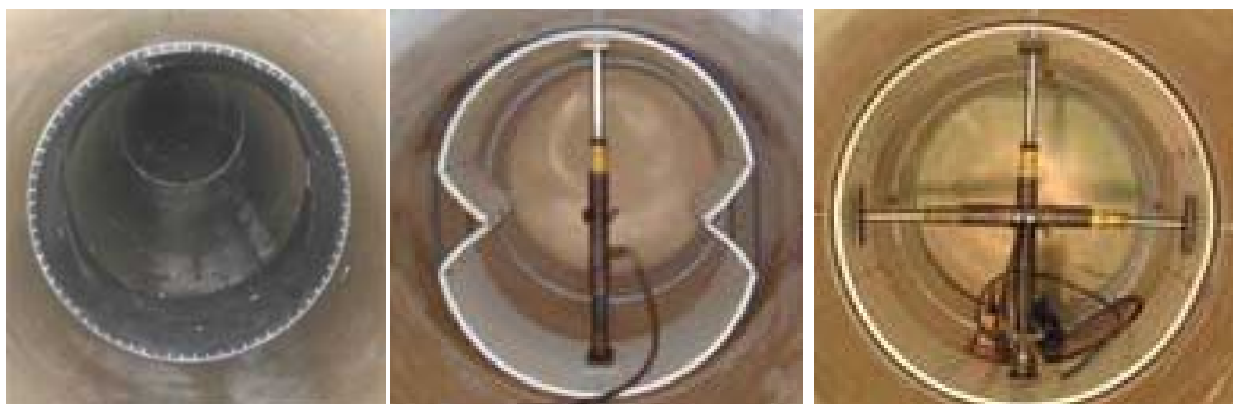
Figure G-7. Examples of Link-Pipe® installation
