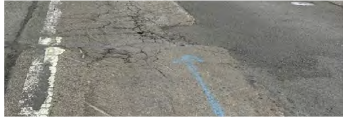
Existing pavement and waterline trench patch on Molalla Avenue
