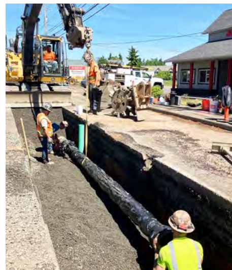
Shared Trench: 30-inch and 8-inch water mains
