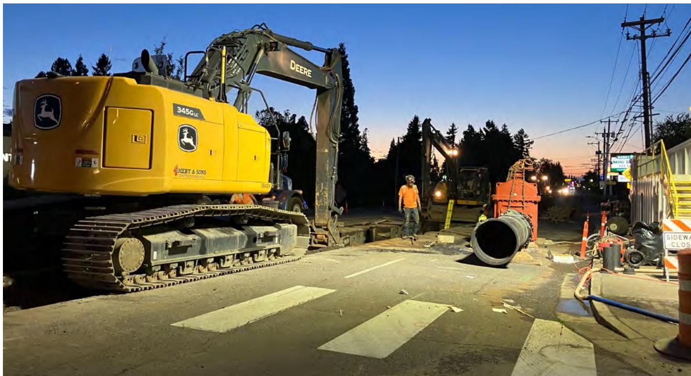
Night Work at Warner Milne & Molalla Ave. 30-inch gate valve and pipe
