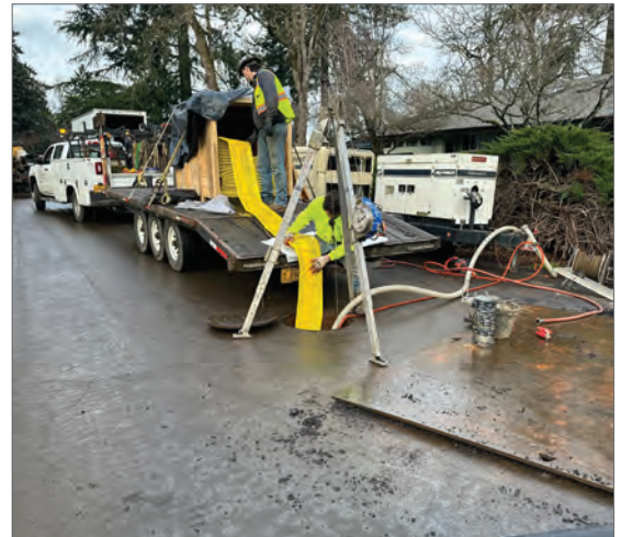
CIPP lining of mainline sewer pipe
